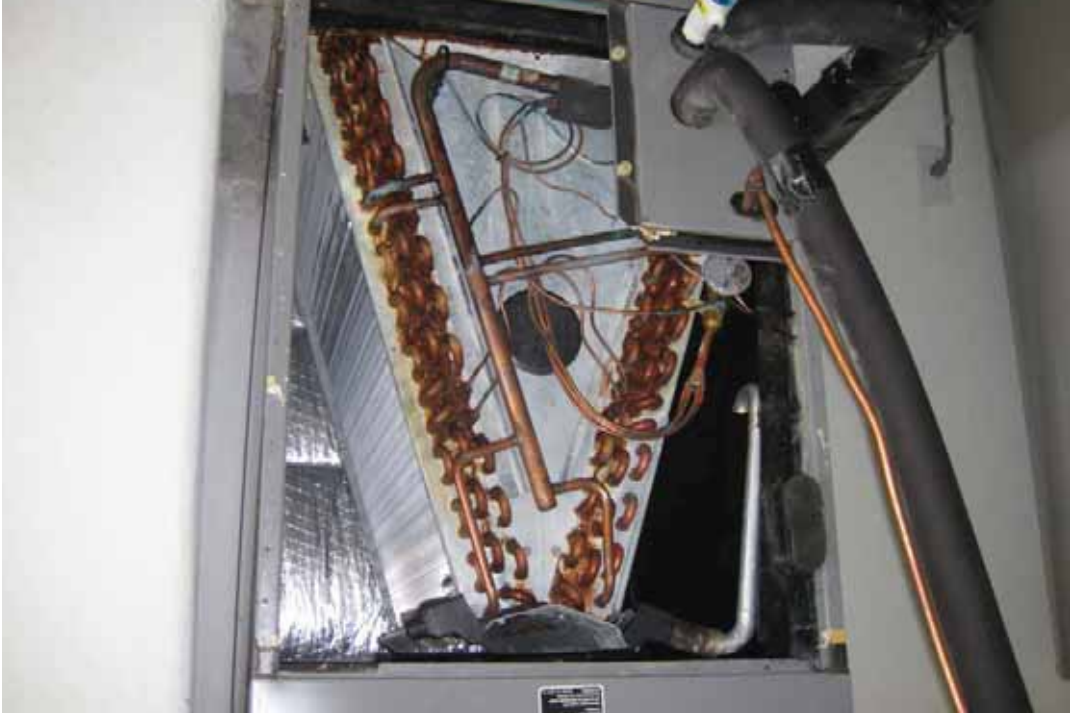
Air Conditioning Evaporator Coils from Home without Chinese Drywall
