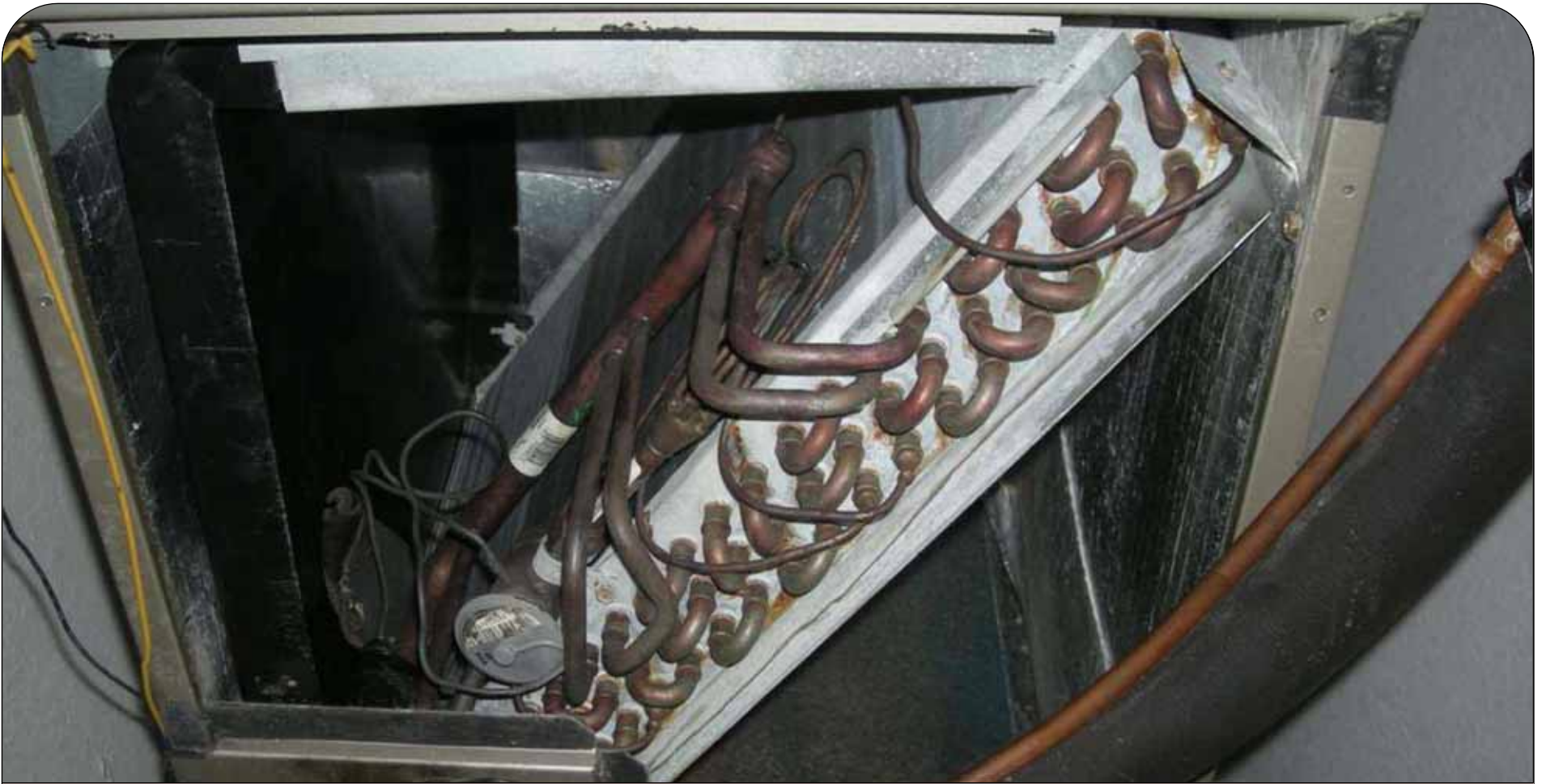
Mild corrosion
