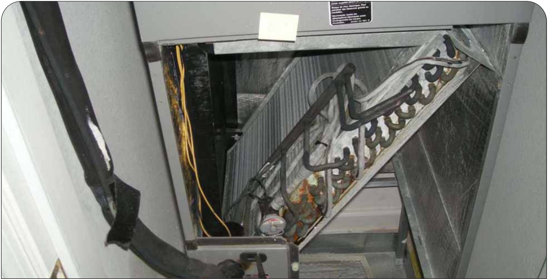
Corroded coil
