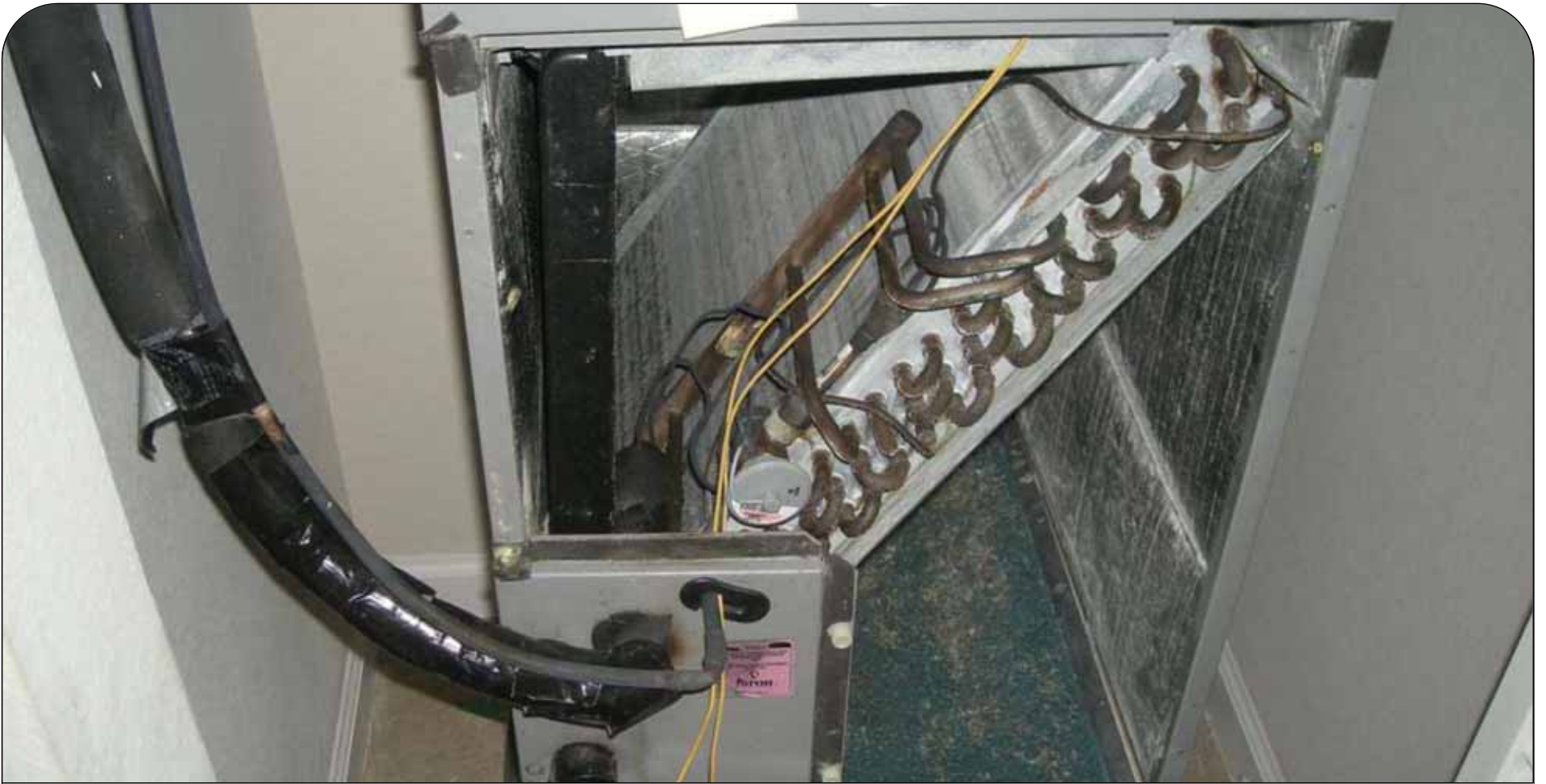
Corroded coil
