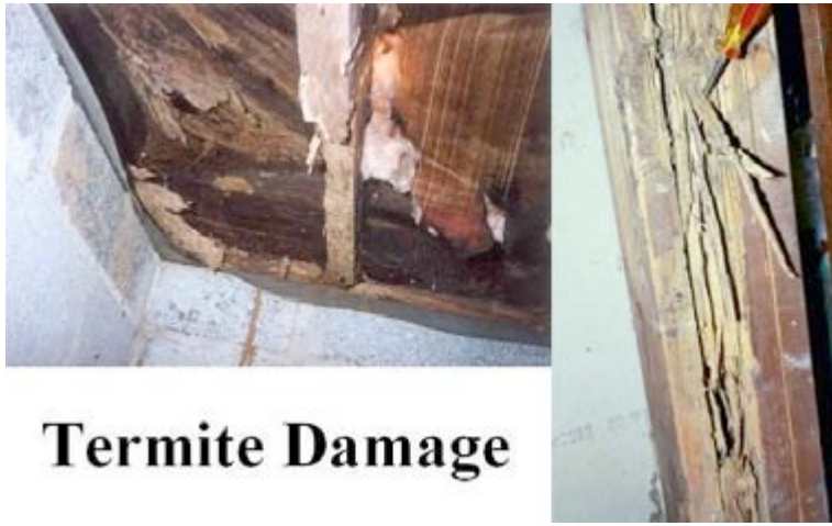
Figure 29. Termite damage
