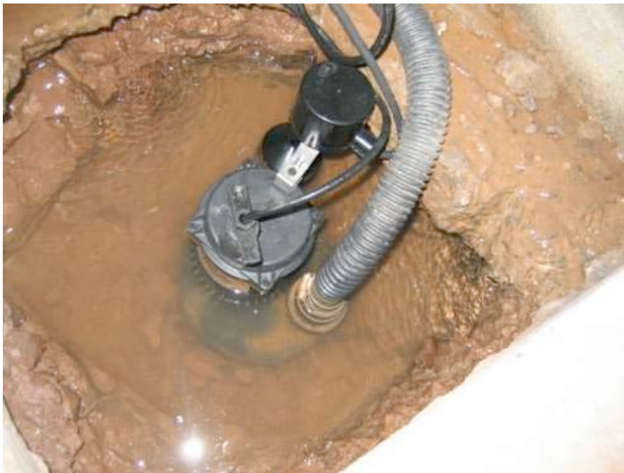
Figure 61. A French drain is a below-grade drainage system that is level with or beneath the basement floor and usually runs around its perimeter. When water gets into the basement, it goes through the French drain and runs into a sump, or sometimes outdoors.
