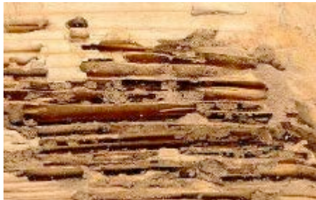
Figure 28. Termite damage
