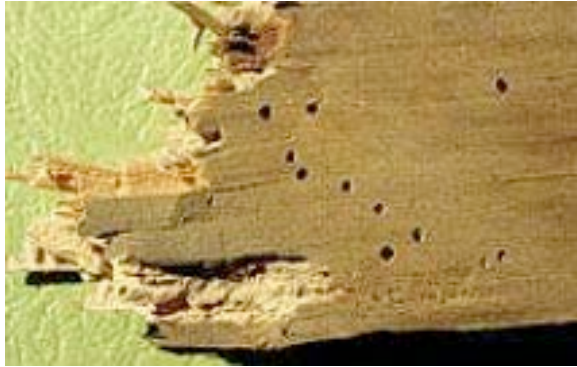
Figure 76. Beetle infestation and damage
