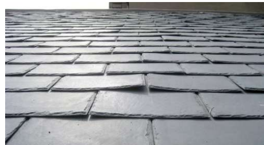
The bowed tiles indicate that this is a composite-slate roof.
