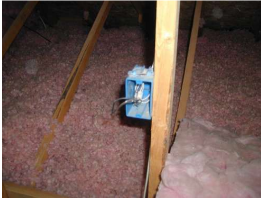
Above: improperly terminated wiring
