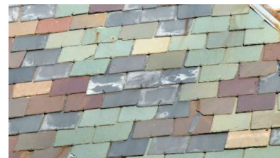
Old slate, like that pictured above, will break when stepped on.
