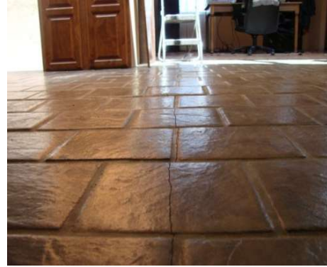
Above: the result of subfloor movement
