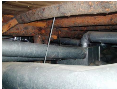
Upper Right: A plumbing distribution pipe is blocking this crawlspace's access hatch.
