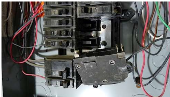
A circuit breaker hangs from its conductor.
