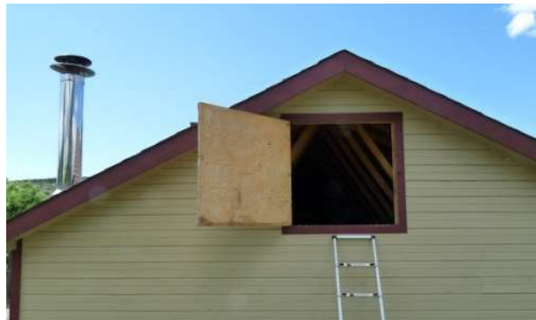
Hatches in gabled ends are best accessed using an extension ladder.
