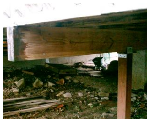
Cantilevered support beam on wooden deck is over-extended, and is sagging. Condition is unsatisfactory, and is indicative of an amateur design and inexperienced installation.
