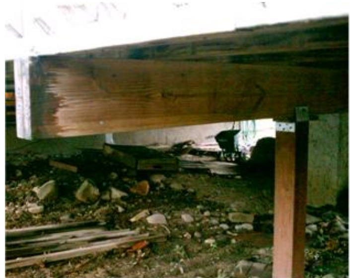
Cantilevered support beam on wooden deck is over-extended, and is sagging. Condition is unsatisfactory, and is indicative of an amateur design and inexperienced installation.
