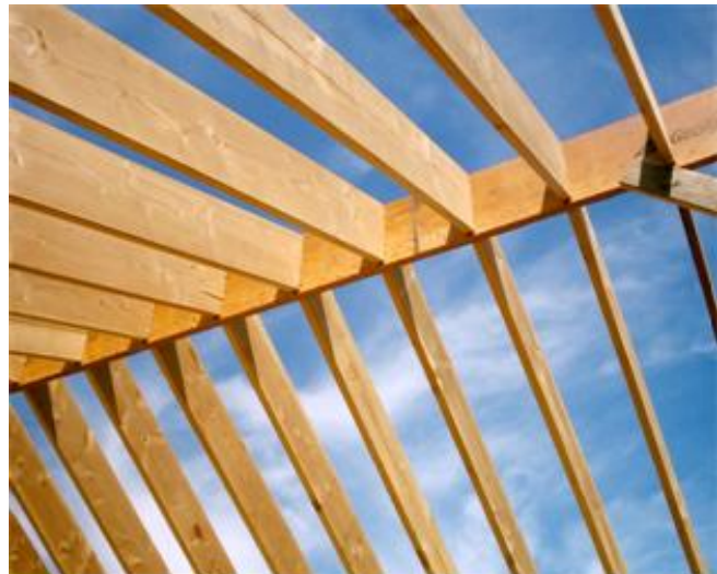
Here's a view of a large, stick-framed roof structure, with ridge beam installed.
