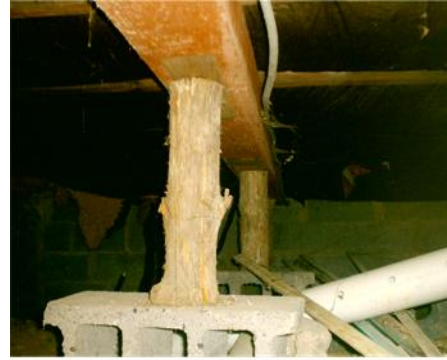
This photo was taken in a crawlspace. Believe it or not, these small tree trunks were all that supported the main girder of an addition.
