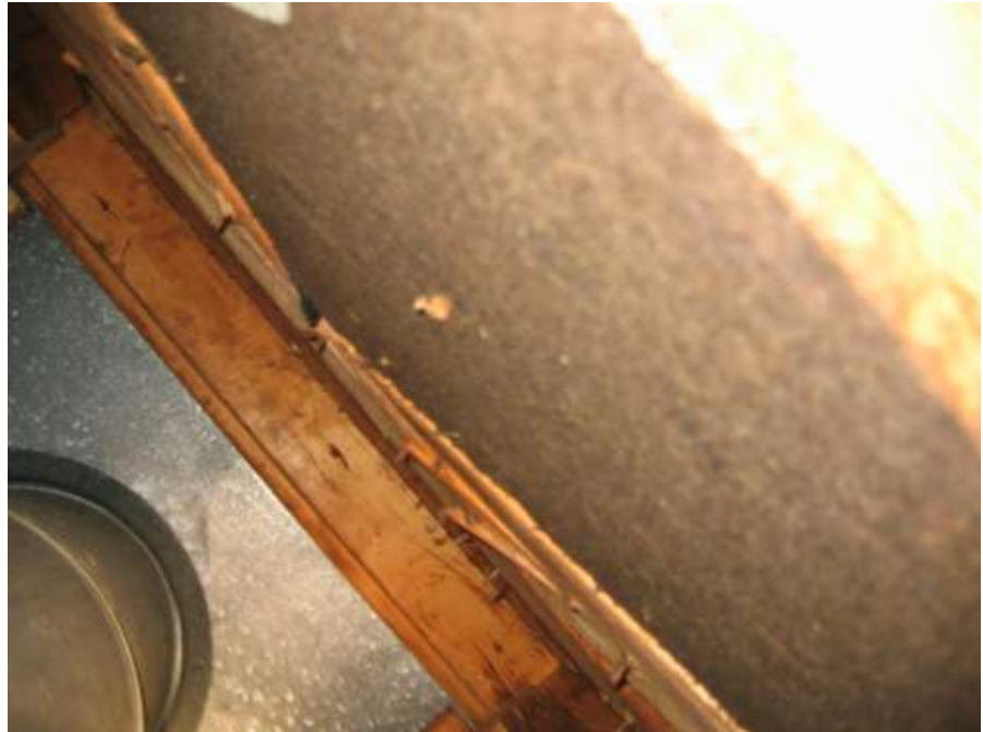
FIRE BLOCKING - CHIMNEY
