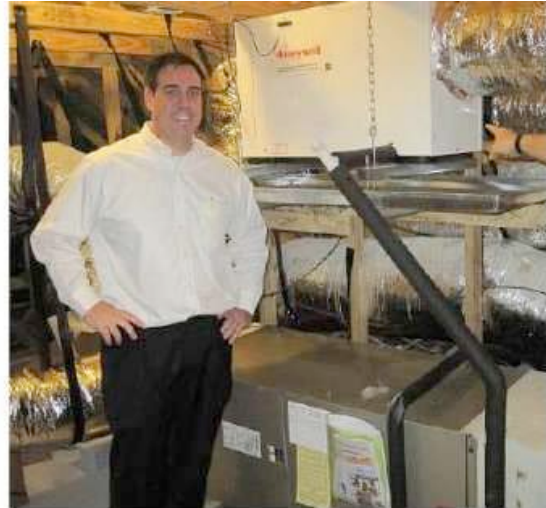
Dehumidifiers can be ducted to a furnace or heat pump central air handler. Dehumidifiers, air handlers, and ducts perform best when installed in conditioned spaces. This dehumidifier and air handler were installed in the insulated attic of a high-performance home built by KB Home in Orlando, Florida (Source: FSEC).
