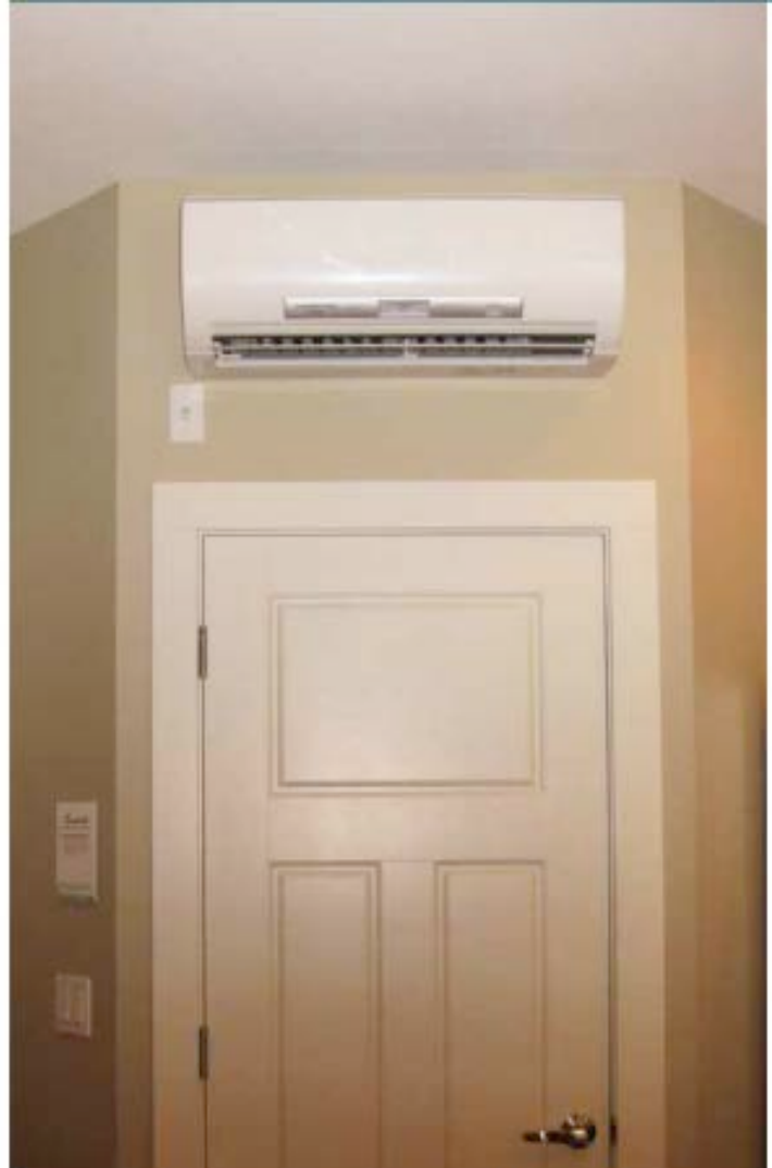
Ductless heat pumps can provide efficient zoned heating and cooling.
