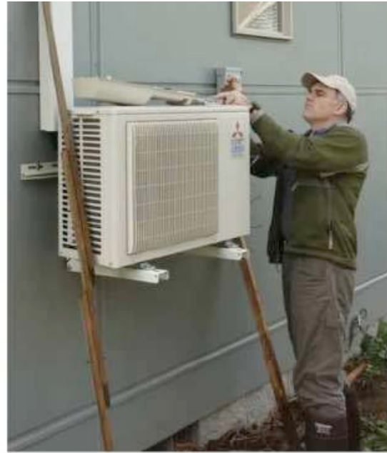
Ductless heat pumps are sometimes referred to as mini-splits because they have a single outdoor unit and one or more small, wall-mounted indoor air handler units. The outdoor unit can be located on a concrete pad or mounted on an exterior wall (Source: Northwest Energy Works).
