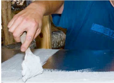
Mastic is a thick sealant that is painted on to rigid ducts to seal seams and joints (Source: FSEC).
