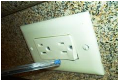
above: a melted outlet
