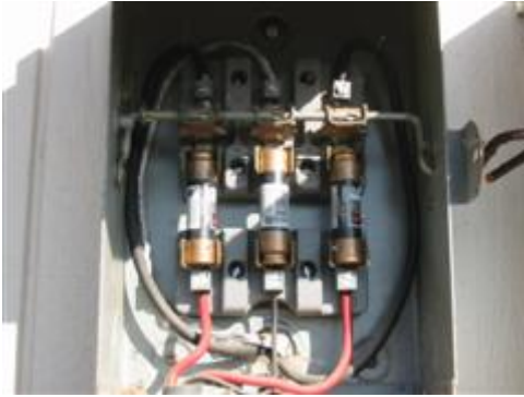
Above left: fused neutral main disconnect ( courtesy of Pat Dacey ); Above-right: fused neutral load center ( Photo courtesy of Jeff Pope )
