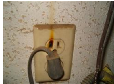
above: an outlet displaying signs of arcing
