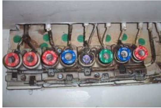
Above left: fused neutral main disconnect ( courtesy of Pat Dacey ); Above-right: fused neutral load center ( Photo courtesy of Jeff Pope )
