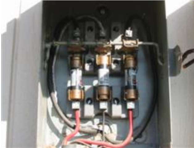
above left: fused neutral main disconnect ( courtesy of Pat Dacey ); above-right: fused neutral load center ( Photo courtesy of Jeff Pope )
