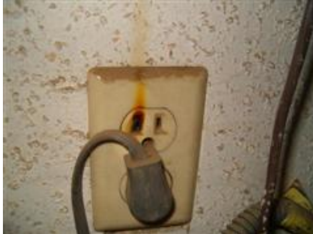
above: an outlet displaying signs of arcing
