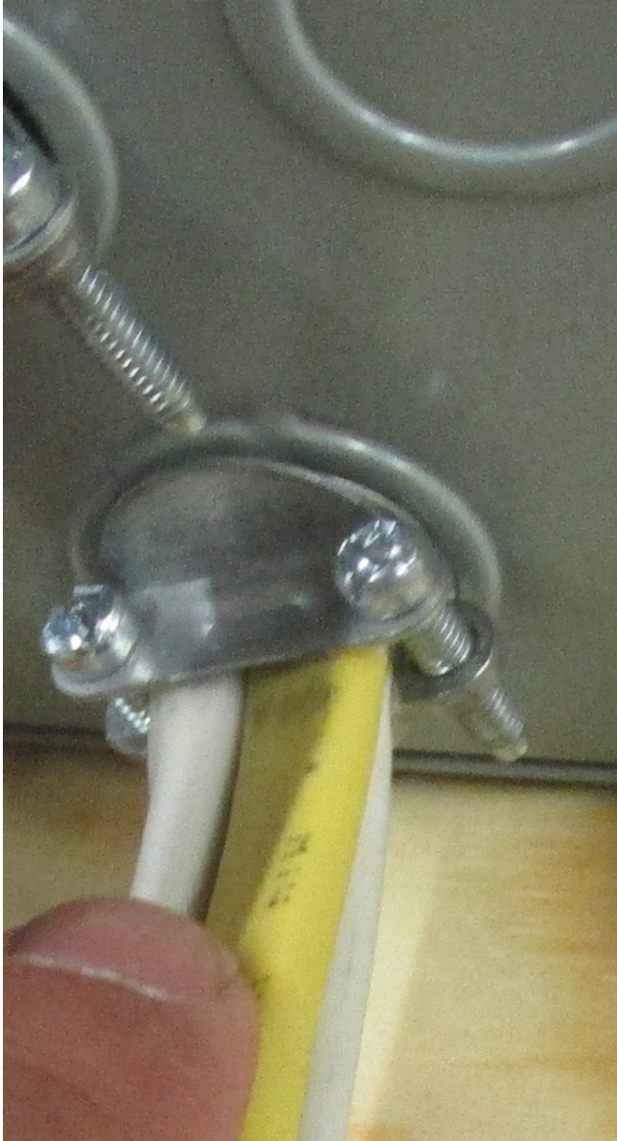
Three cables entering panel through one strain-relief fitting.
