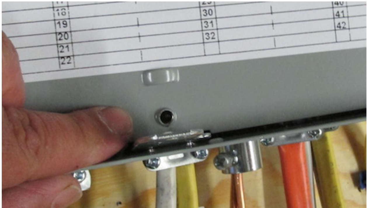
Missing panel cover screw.
