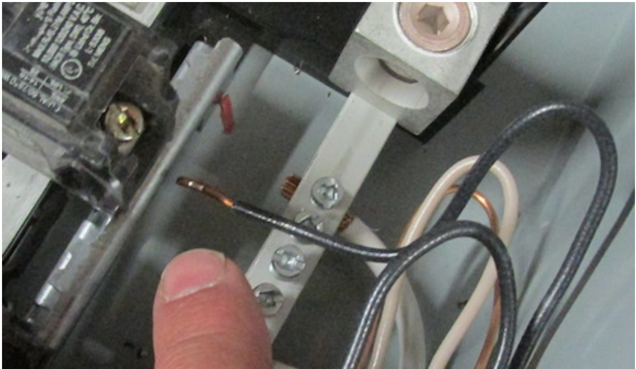
Loose conductor at breaker.
