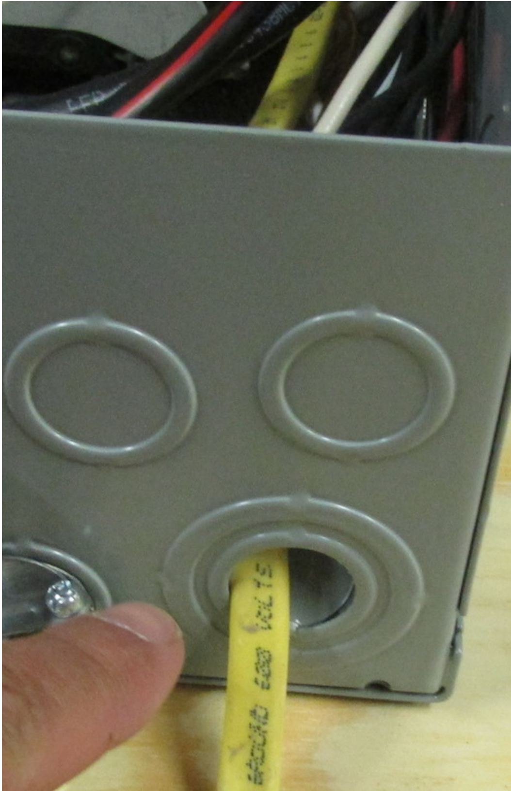
Cable entering panel without strain relief or bushing.
