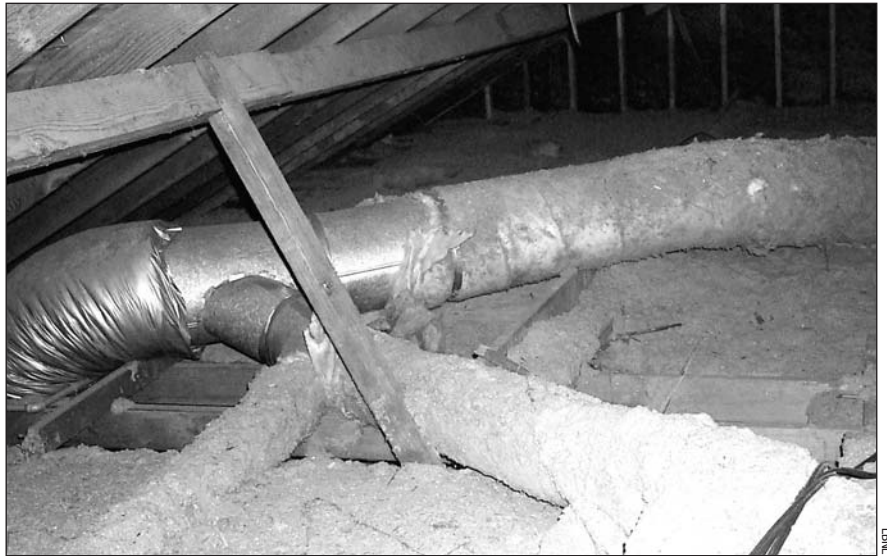
Here we see the poorly insulated sheet metal ducts and blown-in insulation in the attic before the retrofit.
