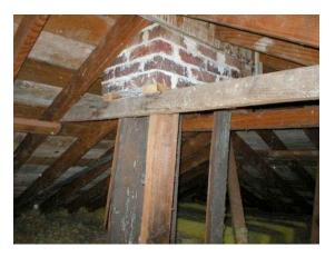
The abandoned chimney might collapse through the ceiling and cause serious or fatal injuries. This is a material defect.
