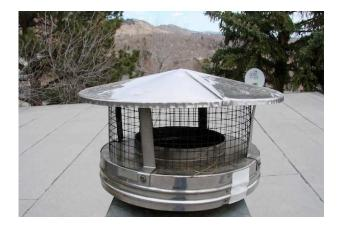
This is a stainless steel spark arrestor. The screen openings should be sized no greater than  $^{1\!/_{\!2}}$  inch.
