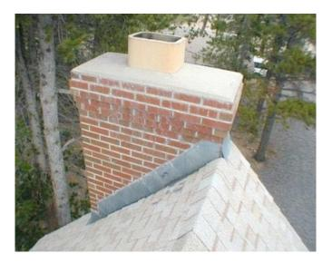
The flashing is improperly installed. The counter flashing is missing.
