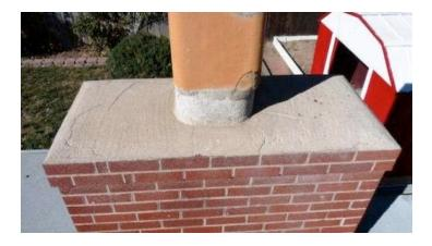
Mortar at the chimney crown is not durable and tends to crack.
