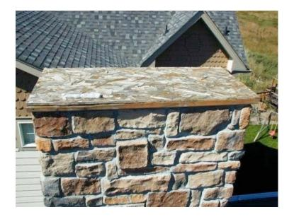
This chimney is missing a cap. Wood must never be used for a crown or cap.
