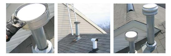
It is a common mistake to apply chimney termination-height requirements (3-2-10 rule) to fuel vents, which cause vents to extend above roofs much higher than needed, in most cases. For example, vent pipes terminating above roof slopes up to 6:12 need to be only 1 foot high.
