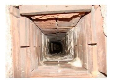
All masonry chimneys must have flue liners installed.
