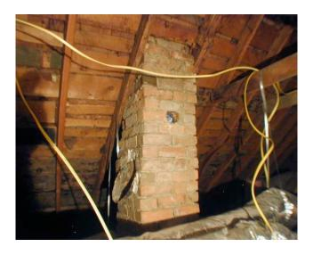
This chimney, observed from the attic space, has an unused opening. This is a fire hazard.
