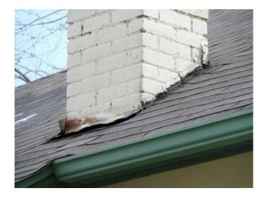
Improperly installed flashing. The flashing is loose and corroded. There is step and counter flashing. The sealant is not permanent.
