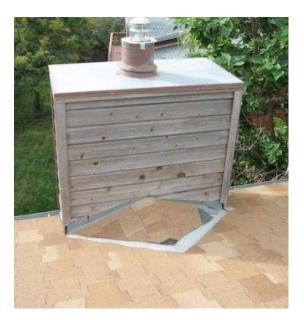
A cricket is a small roof designed to keep water from pooling on the higher-side of the chimney. Framing the cricket will create a couple of little valleys, which need to be flashed correctly.
