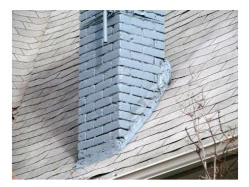
This is incorrectly installed flashing. The step and counter flashing components are missing.
