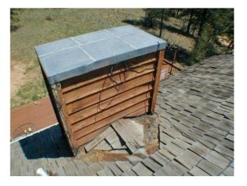
This cricket valley flashing has visible corrosion and accumulated debris. When you see this condition -- and it's common -- scrape away the debris and check the condition of the flashing. Debris will hold moisture against the flashing, and corrosion is likely to advance more quickly in these areas.
