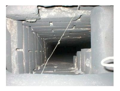
This masonry chimney is missing a flue liner.
