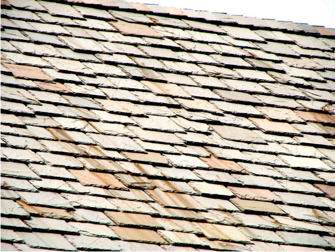
Mineral impurities can cause deterioration in slates.
