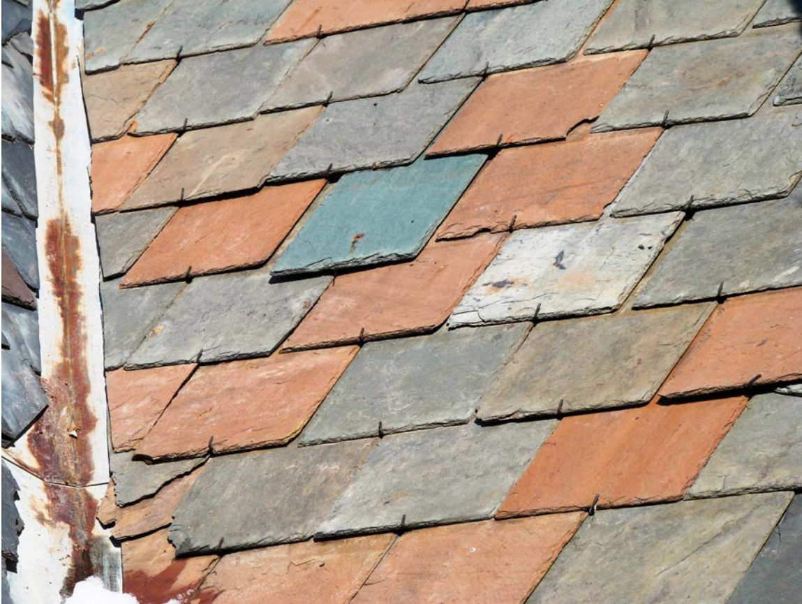
Slate has also been hung from wires.
