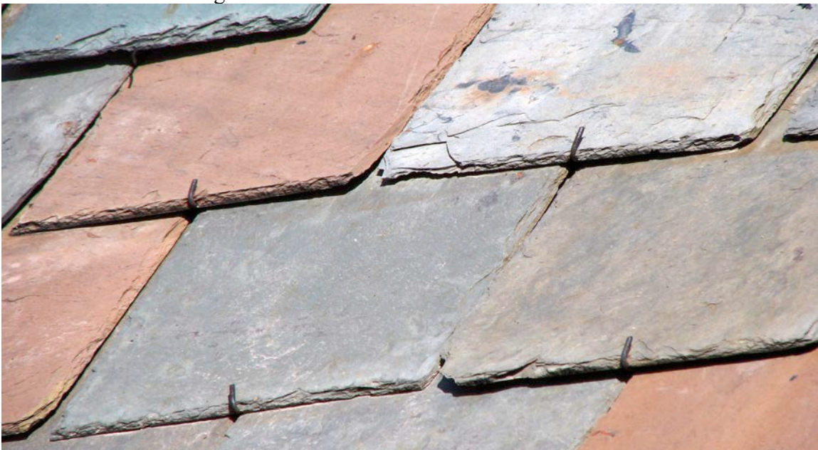
Slate has also been hung from wires.
