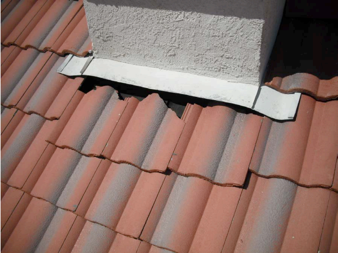
Here the headwall flashing was installed before the tile.
