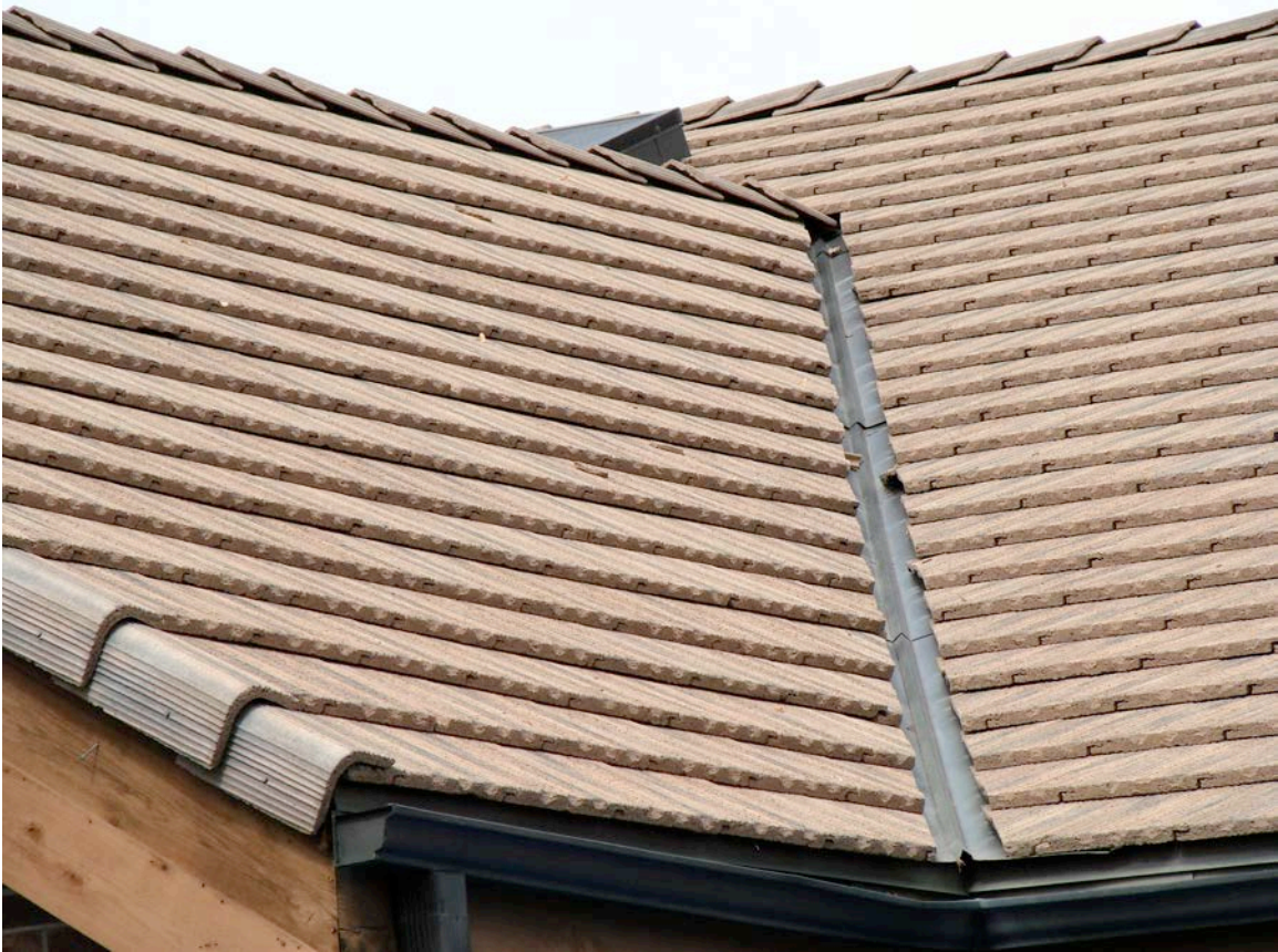
Open valleys will encourage runoff to drain well and help to wash away debris.
