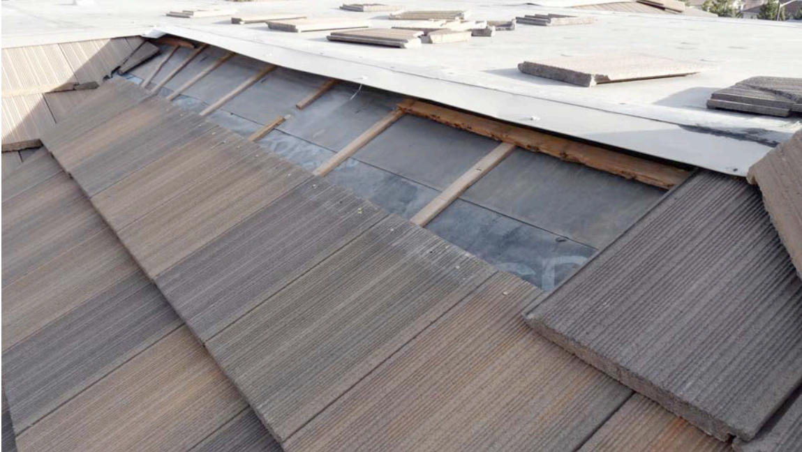
These tiles were held in place using the friction method, which failed in a high wind.
