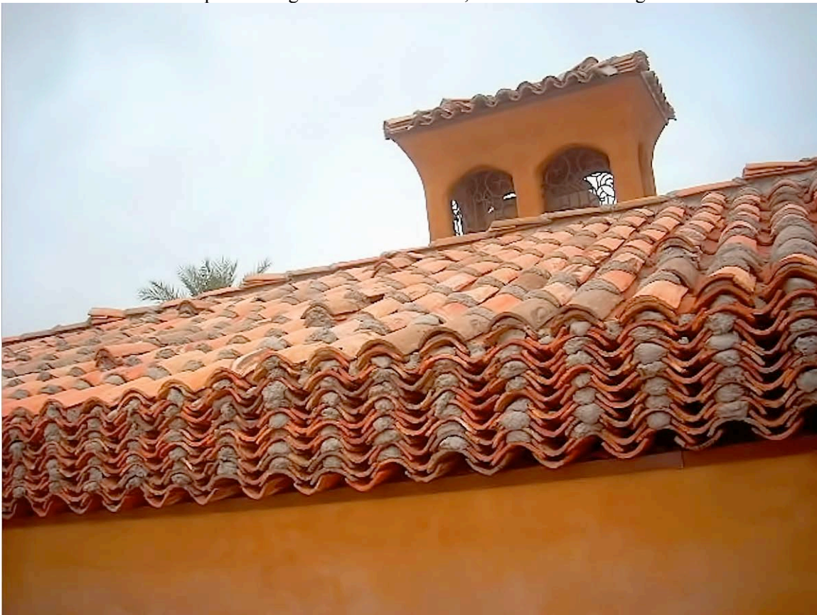
Here's a roof with plenty of mortar. Although this roof is 8 layers thick at the eave, chances are good that it's only one layer thick at the peak. Still, it's heavy, and you'd want to check carefully for sagging of roof framing components like rafters, trusses or sheathing.
