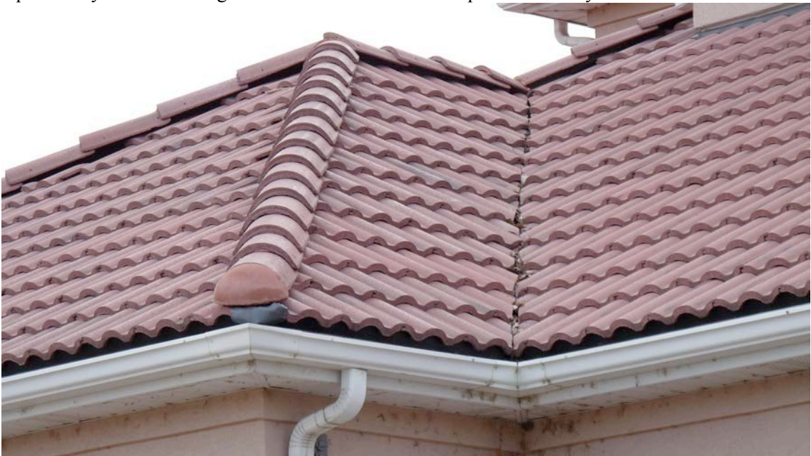
Closed valleys will tend to trap debris, which will accelerate deterioration by holding moisture against the tile.
