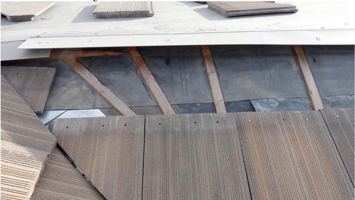
Here the headwall flashing was installed before the tile.
